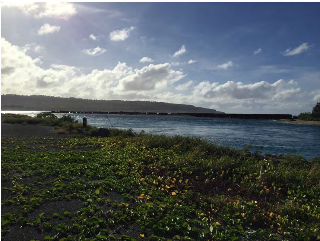
Tinian Harbor Main Breakwater
